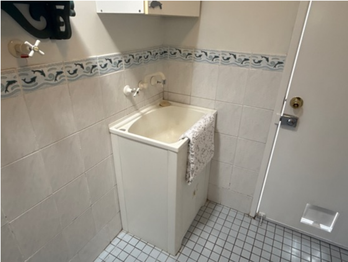
Water pressure tested, is sufficient - the tub displays low level wear, consistent with age.
