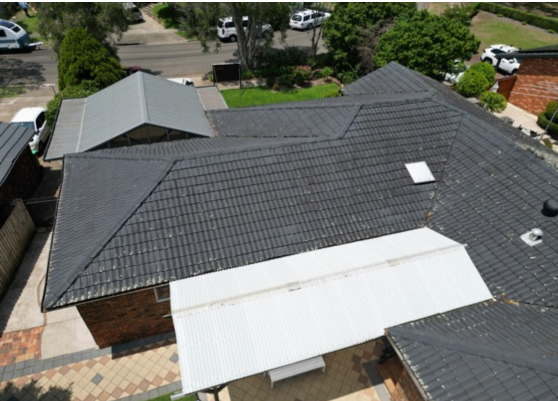
Rear sheet metal roof sheets present in satisfactory condition.
