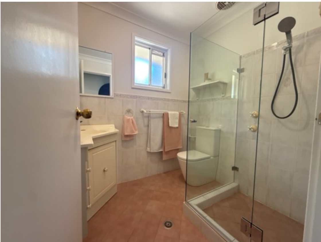
The ensuite bathroom area tested for leaks, fixings and stability was all clear at the time of inspection.
