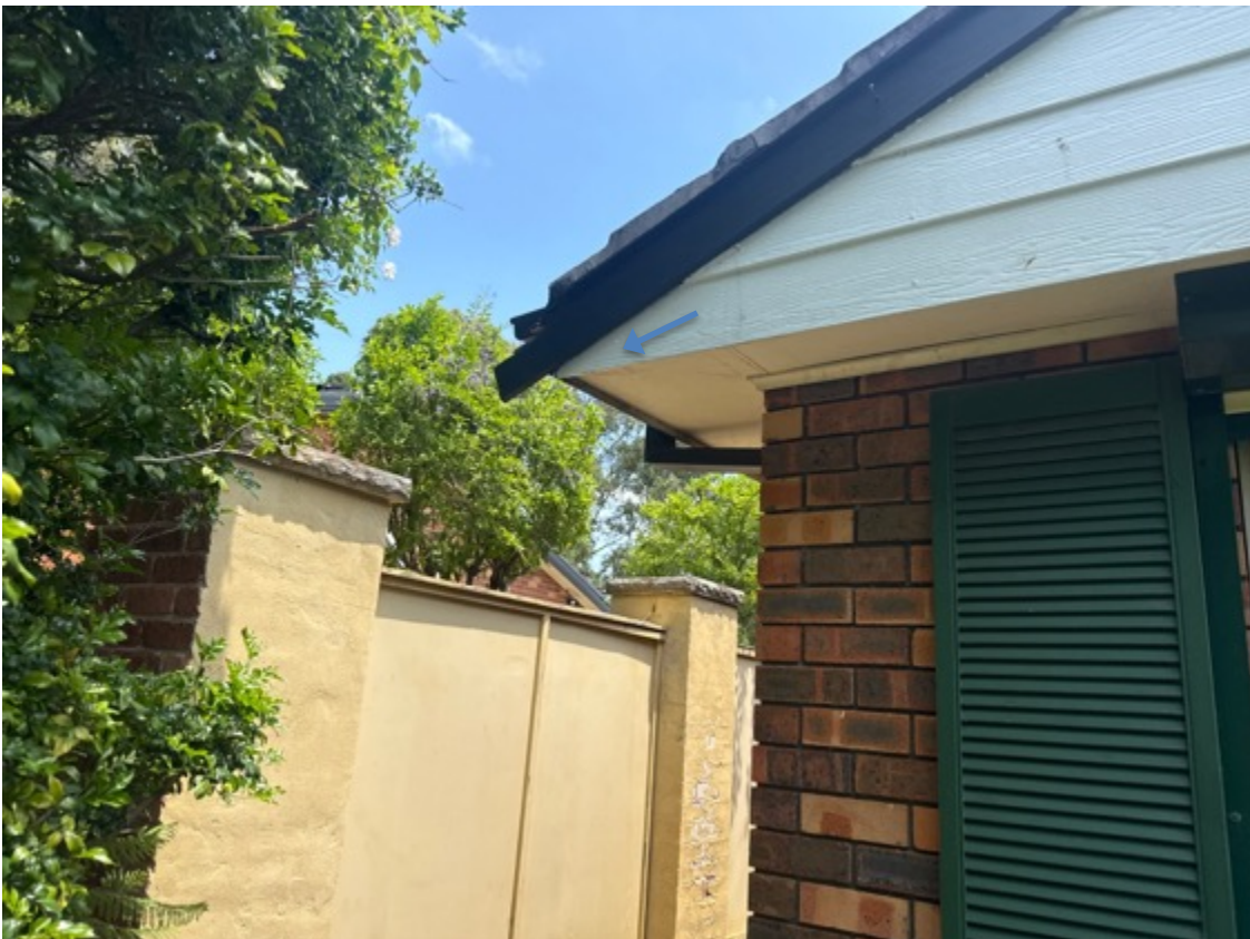
Exterior timber displays moderate level weathering - consistent with age.
