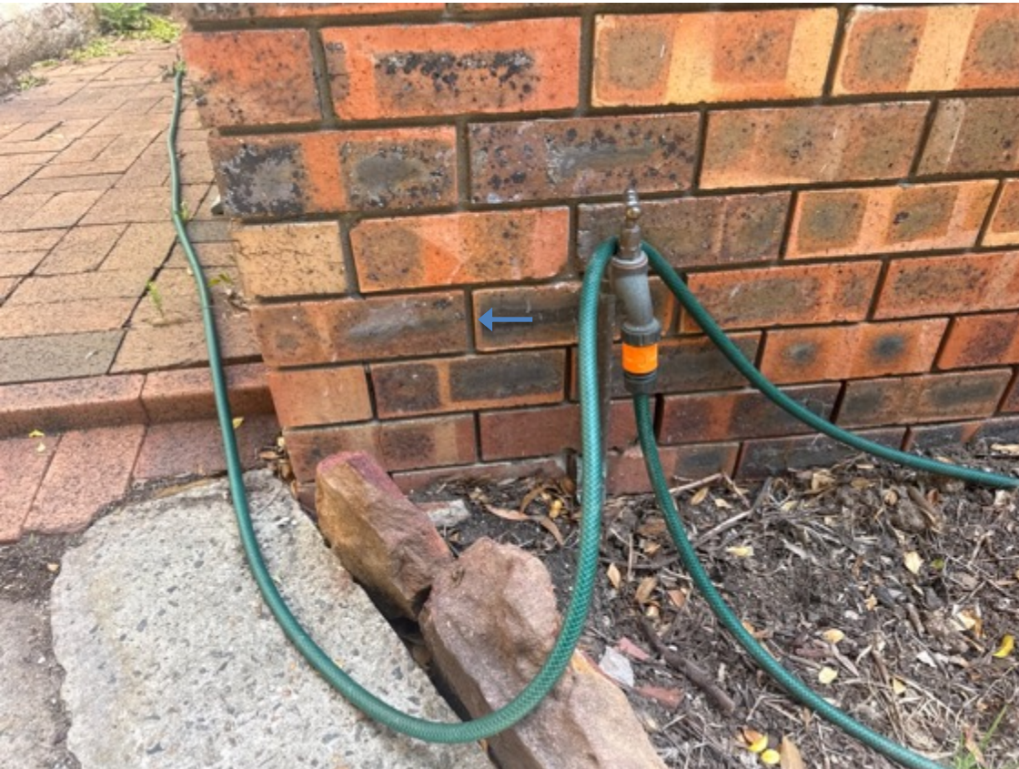
Isolated sections of external brickwork displays category one cracking (front left elevation example above.)
