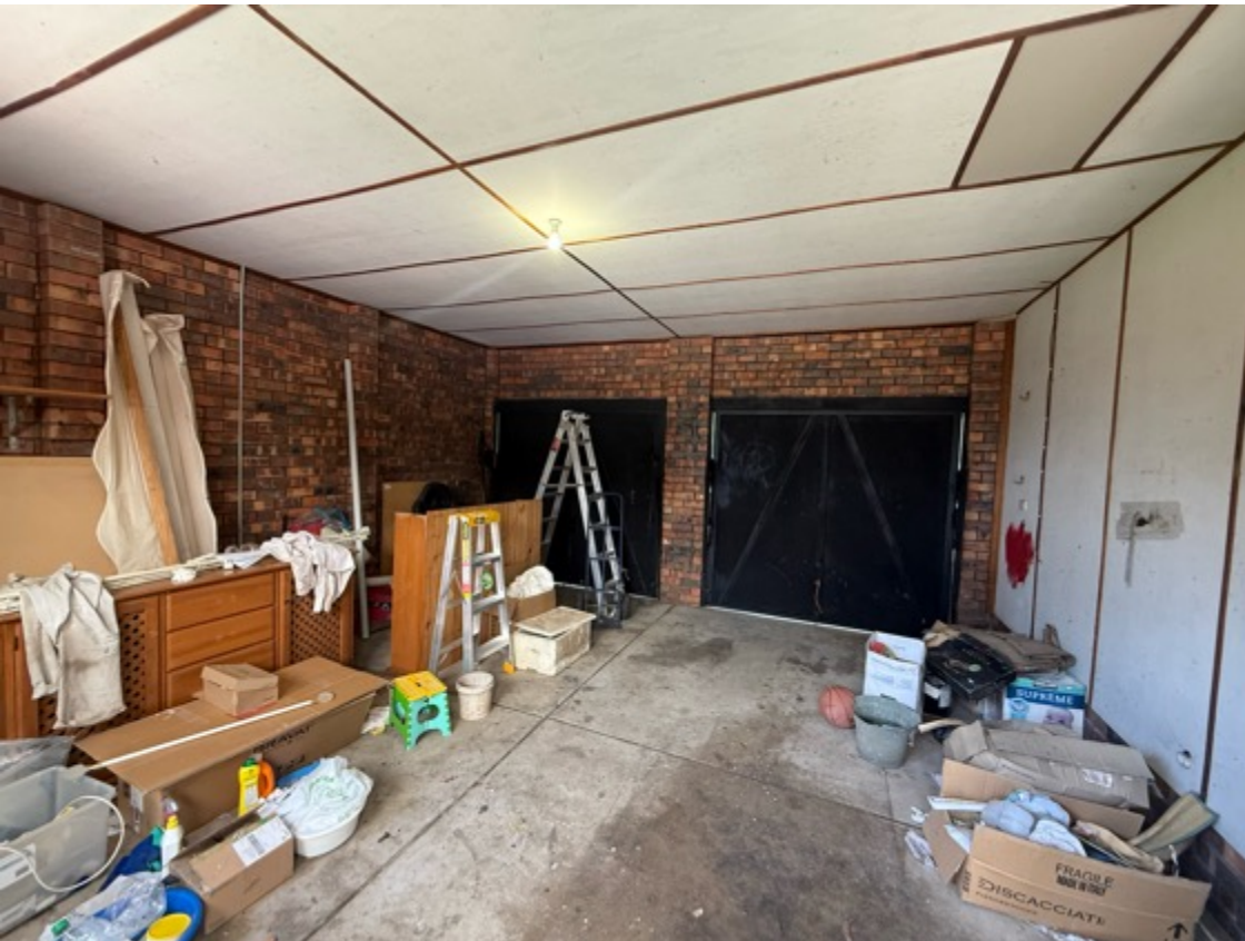
The garage area is in serviceable condition.
