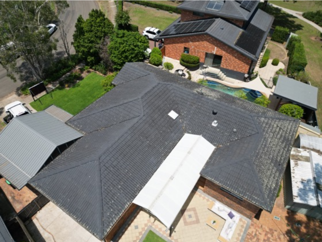
The roof exterior presents in satisfactory condition for the age.
