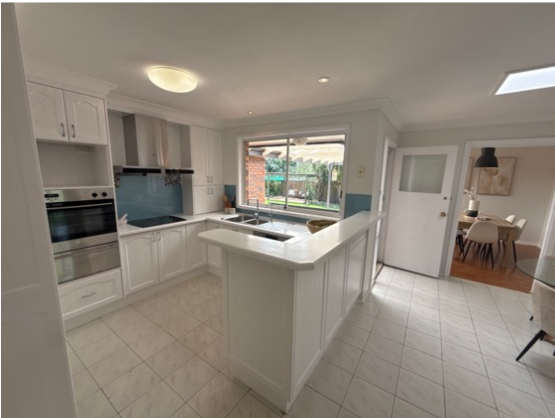
The kitchen area presents in satisfactory condition for the age.
