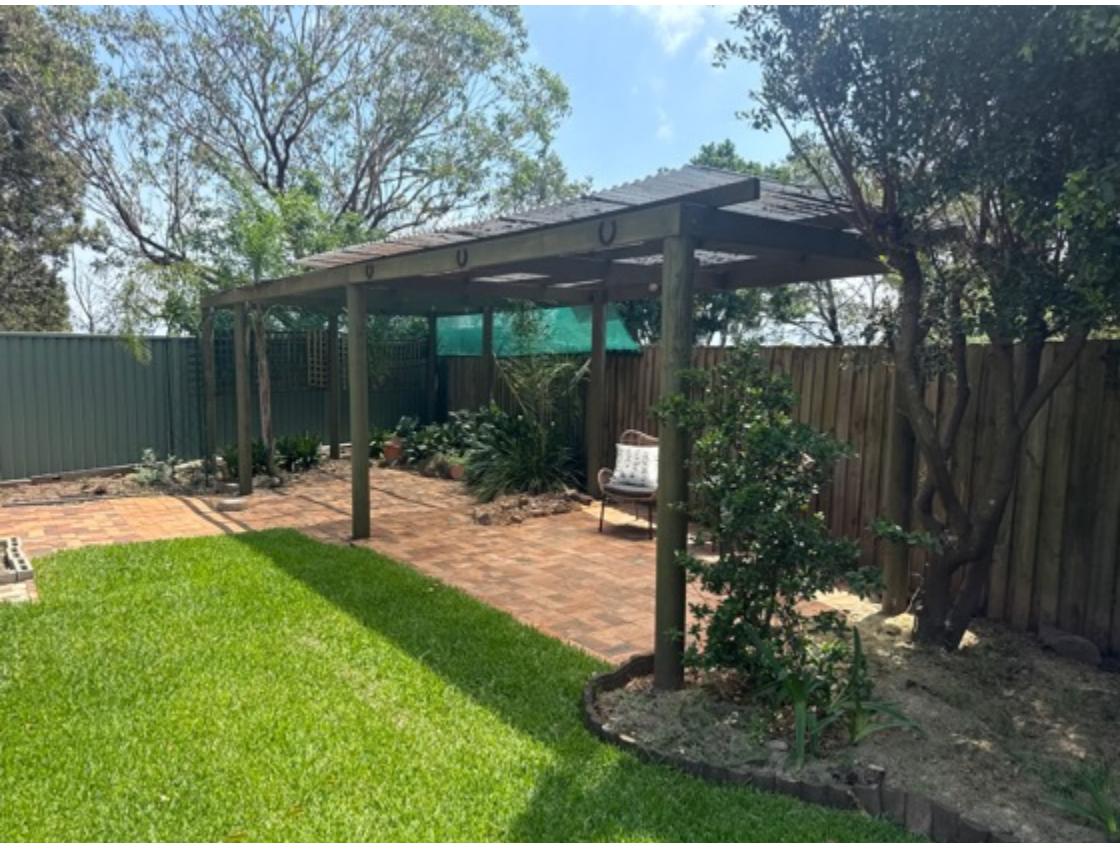
The rear pergola checked is structurally sound.
