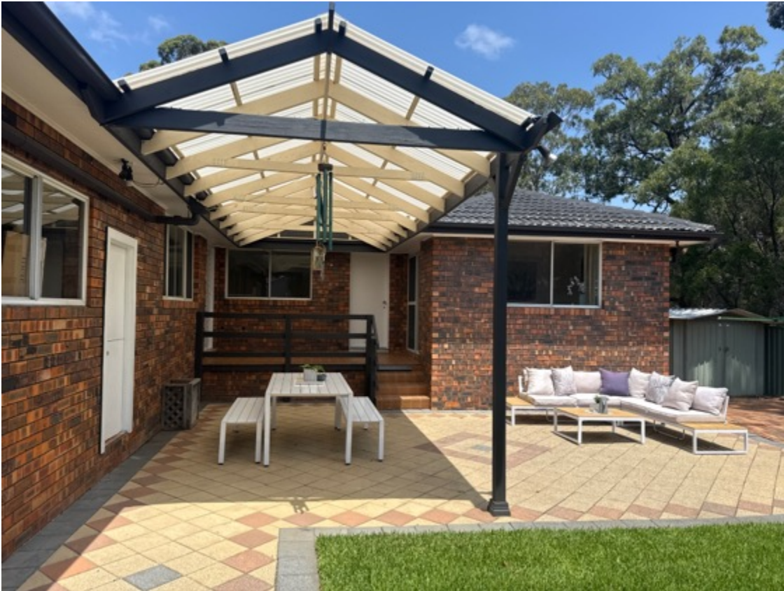
The rear pergola checked is structurally sound.
