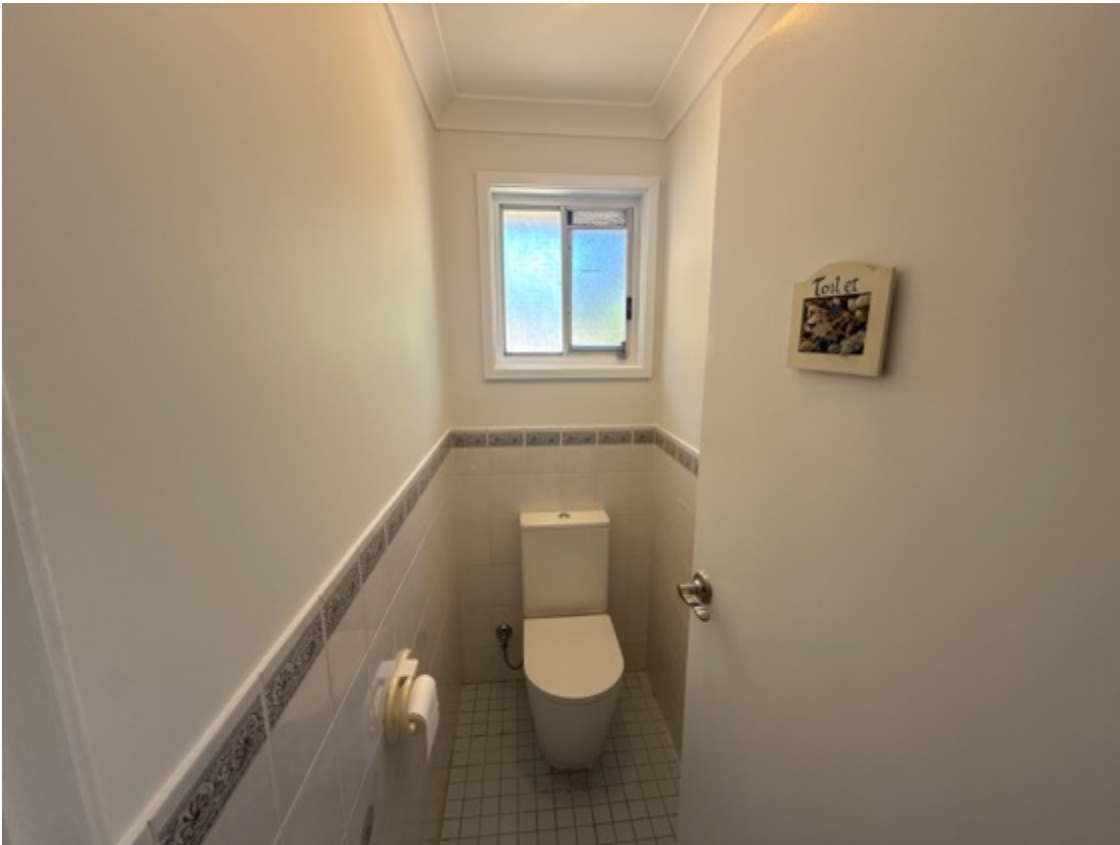
The common toilet tested, functioned at the time of inspection.
